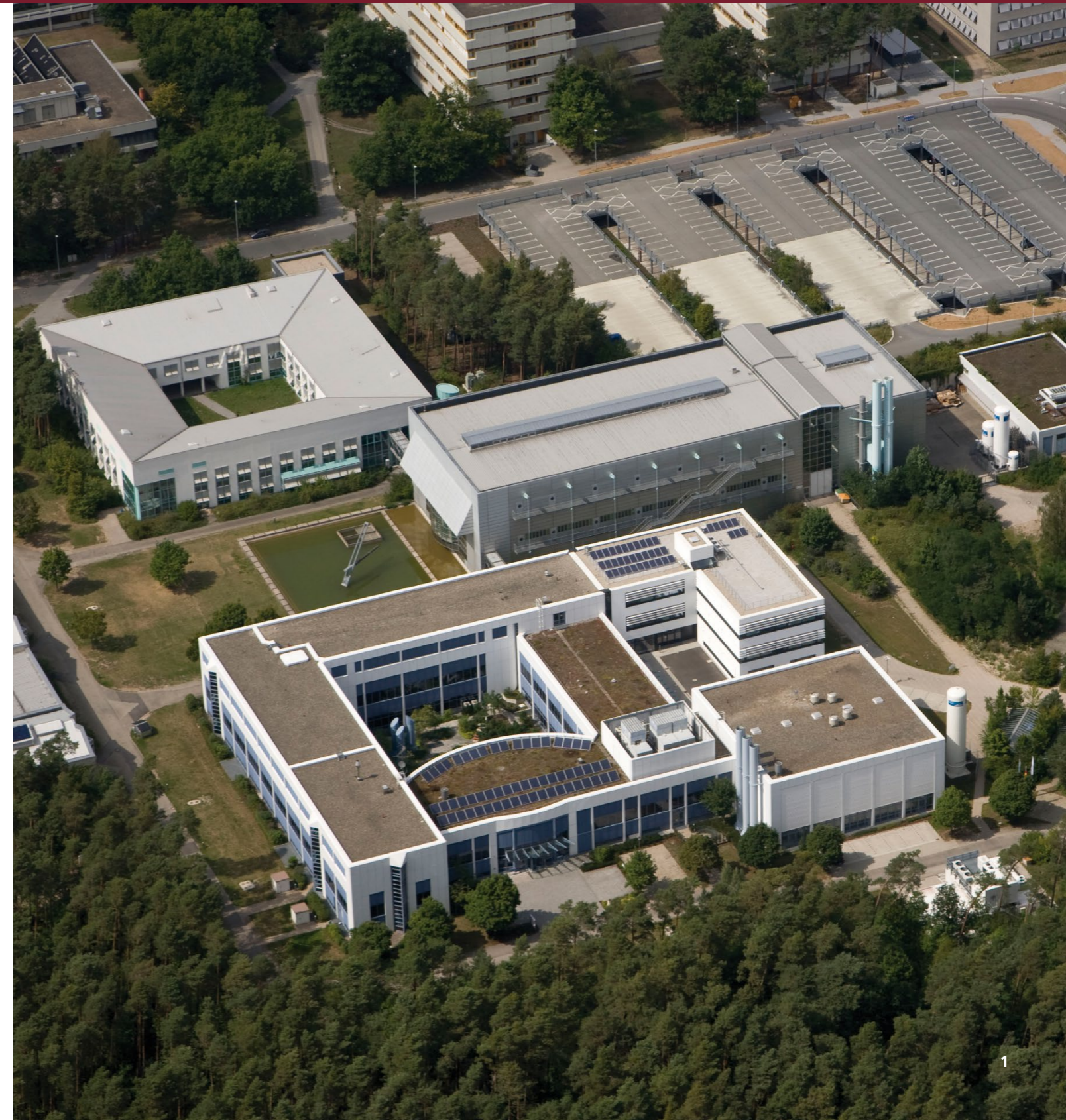
1 Building of the Fraunhofer IISB with test center for electric vehicles, cleanroom, and new laboratory building; behind: cleanroom laboratory and building of the Chair of Electron Devices of the University of Erlangen-Nuremberg. Image: Kurt Fuchs / Fraunhofer IISB
